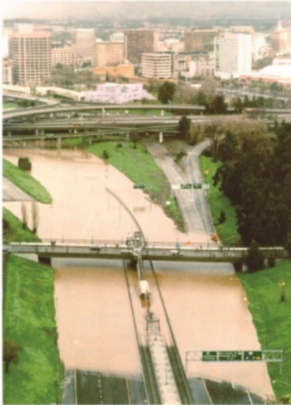
Figure 3. Major inundation from the flood of 1995 occurred on Highway 87 in San Jose's downtown area
